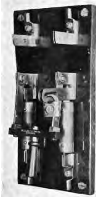
Fig. 1. Switch with Locking Device.
